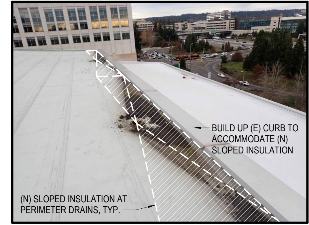
NEW SLOPED INSULATION AT MECHANICAL WELL (BID ALT)
