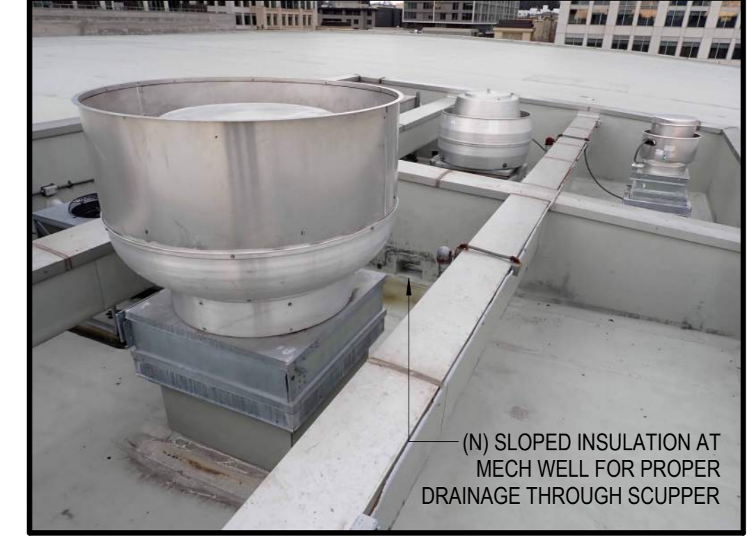
NEW SLOPED INSULATION AT MECHANICAL WELL (BID ALT)
